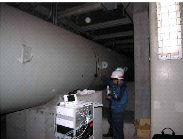
Figure 12 Overview of measurement test at a sea circulation water pipe in a fossil-fired power station.
