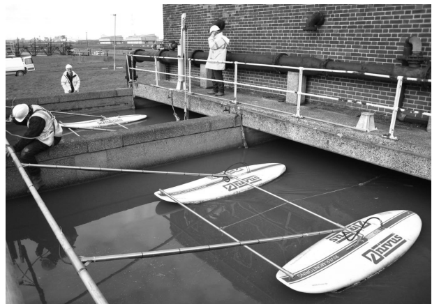
Figure 6: Float system by use of surf boards
