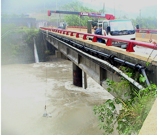
Figure 2: ADP and sounding hanged by a crane for measuring velocity distribution.
